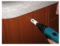
Using a 2½" screw, fasten the lower backet to siding making sure bracket is level with bartop. Using a 1/8" drill bit, drill other side upper mounting hole.
