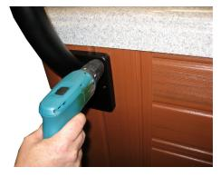
Fasten 2½" screw to other upper mounting hole. Pre-drill and fasten the other four screws. Once the lower bracket has been installed, remove the 6 screws and remove bracket from the spa.
