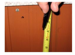
Using a 1/8" drill bit, drill designated upper mounting hole. Using a 1" hole saw, drill center hole.
